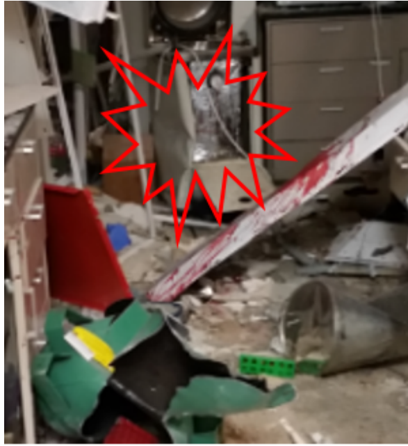
Figure 12: Autoclave impact damage from the smaller tank piece
